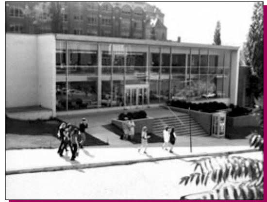
The Library with the addition that was completed in 1962. This is now where the Law School is located.
