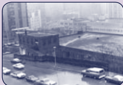
Geyer Garage formed the foundation for the new library construction in the 1970s.
